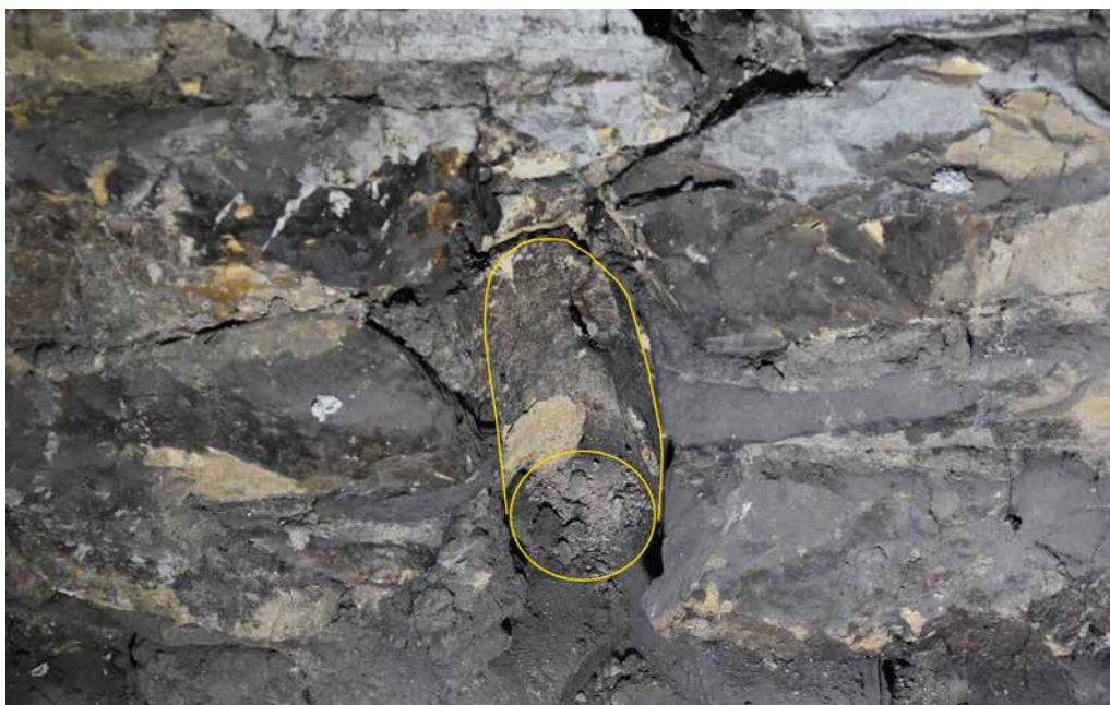
Fig. 15. St. Agnes Monastery, attic of the presbytery of the Church of St. Francis. One of the two sockets of wooden logs in the axial field of the polygon of the presbytery (photo by the author, 2024).
