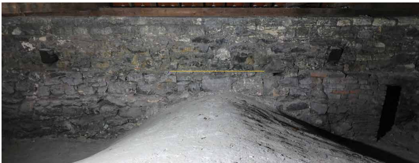
Fig. 11. St. Agnes Monastery, attic of the presbytery of the Church of St. Francis. The top of the vault and the layer A from the first building phase (1238–1245), the bedding joint of layer B from the reconstruction of the timber reinforcement from after 1300 marked in yellow (photo by the author, 2024).
