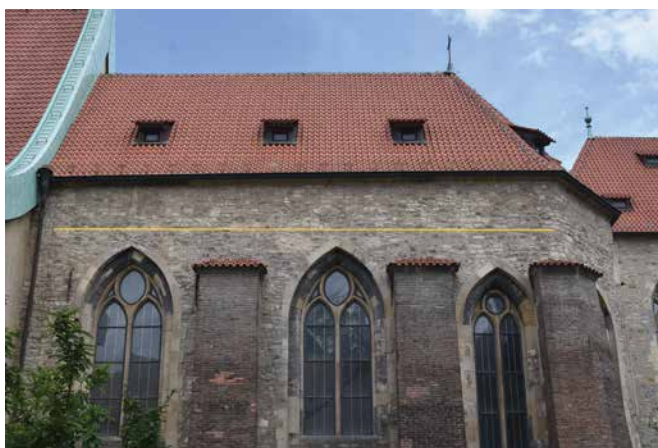
Fig. 6. St. Agnes Monastery, presbytery of the Church of St. Francis. View from the south showing the break between the first building phase and the post-1300 one. Above the window reveals a horizontal break (highlighted in yellow ) between the older masonry and the layer B masonry containing timber reinforcement (photo by the author, 2024).
