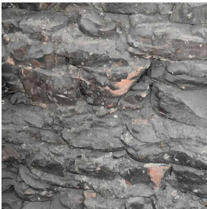
Fig. 13. St. Agnes Monastery, attic of the presbytery of the Church of St. Francis. The pinkish colour of the stone blocks in layer A shows that this layer was damaged by fire (photo by the author, 2024).
