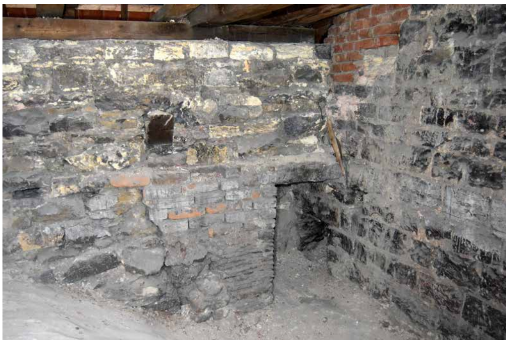
Fig. 7. St. Agnes Monastery, presbytery of the Church of St. Francis. View of the south-west corner of the attic at the junction of the southern outer wall of the presbytery made of roughly shaped stone and the eastern gable of the nave of the church of St. Francis made of regular stone blocks from the 1230s (photo by the author, 2024).
