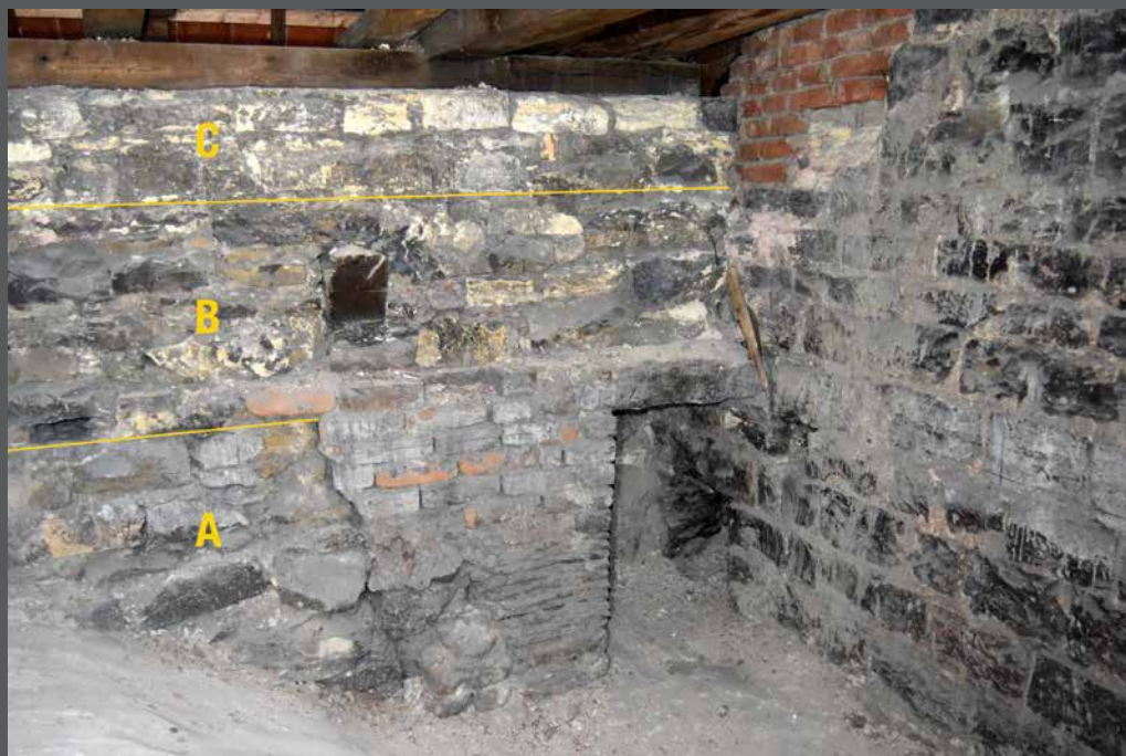
Fig. 9. The same view as in Fig. 7 with the interface between phases A , B and C marked (photo und designation by the author, 2024).
