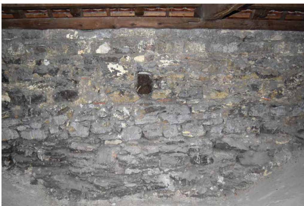
Fig. 8. St. Agnes Monastery, attic of the presbytery of the Church of St. Francis. The face of the south outer wall above the vaults with the cut-off remnant of the timber clamp (photo unedited).
