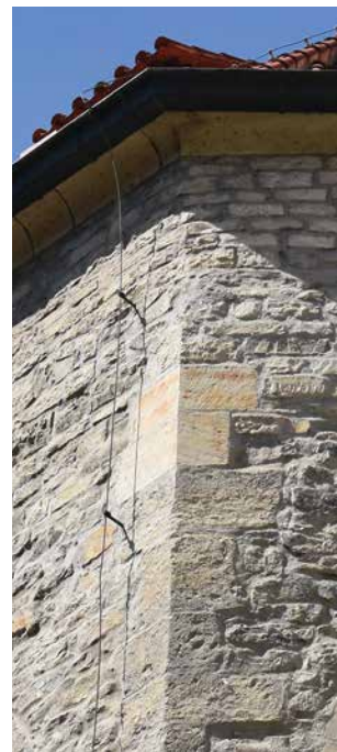
Fig. 5. St. Agnes Monastery. View from the east of the presbytery of the church of St. Francis ( left ), showing the break between the first building phase (1238–1245) and the post-1300 one, evident not only in the structure of the masonry, but also defined by the ashlar quoins (see Detail). The northern part of the presbytery is covered by the buttress of the Church of the Holy Saviour (photo by the author, 2024).
